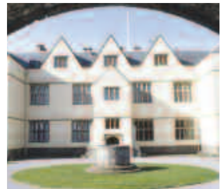
Exterior view of St Fagans Castle (built circa 1590). Electric under-floor heating was introduced into the kitchen in 1991.
