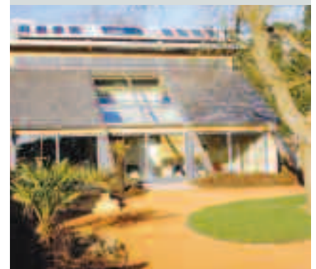
Y Tŷ Gwyrdd (a 'House for the Future') designed by Jesticoe & Whiles and built at the Museum in 2001. A ground source heat pump is one of four different systems available for heating the interior.
