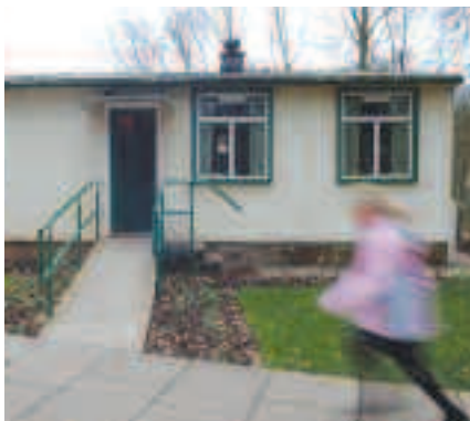
Aluminium prefab: moved to the Museum in 1998. An electric under-floor heating system was installed in order to maintain even temperatures throughout the building.
