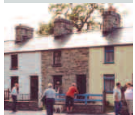
Fron Haul: a terrace of four houses moved from Tanygrisiau, Gwynedd, and re-erected at the National Slate Museum, Llanberis in 1998. Electric under-floor heating was incorporated in the houses, the slate-flag floors acting as heat reservoirs, enabling a constant background temperature to be maintained even at nights and in winter.
