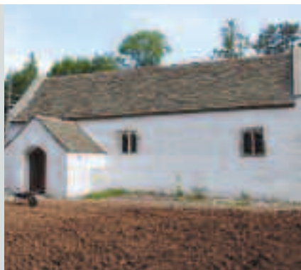
St Teilo's church: rebuilt at the Museum to its appearance circa 1520. A ground source heat pump has been incorporated to improve inside temperatures and humidity levels.
